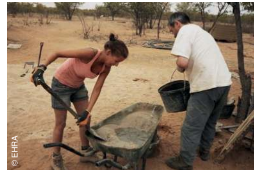
Mix 1 spade cement + 4 spade of sand + water.
